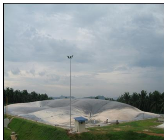
Ponding system for palm oil mill effluent (POME) treatment and covered lagoon technology
