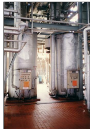
Figure 2 : Floating top closed anaerobic digester at KS
