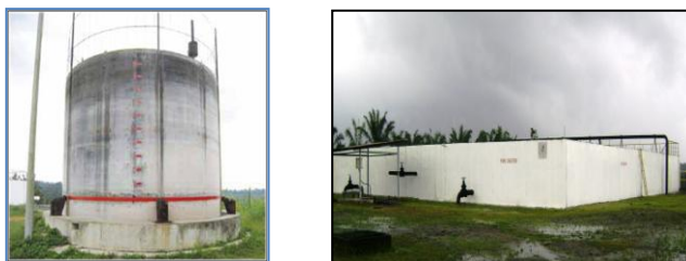
Figure 1. Biogas storage tank and high efficient methane fermentation system
