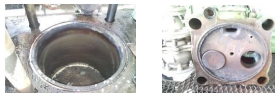
Figure 2. Condition of the combustion chamber of a gas generator using biogas for > 10000 h
