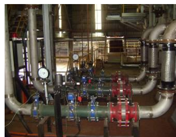
Figure 3: 3 x 100 m 3 /hr biogas burner and flaring unit installed at the mill
