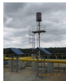
Figure 3: 3 x 100 m 3 /hr biogas burner and flaring unit installed at the mill
