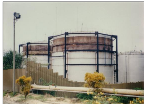
Figure 2 : Floating top closed anaerobic digester at KS
