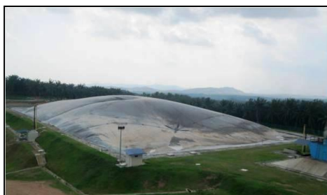
Figure 1: Covered lagoon biodigester installed at the mill
